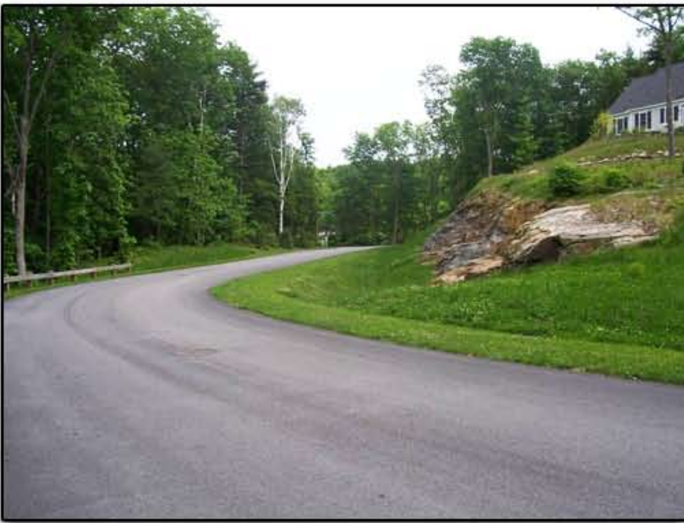
Looking East toward Pine Hill Road
