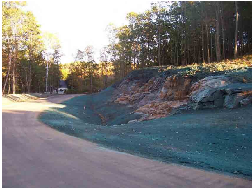
Looking East toward Pine Hill Road, 10-7-2006
